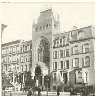
The Church of the Heavenly Rest.
